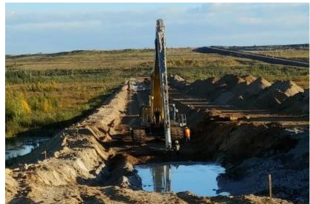
Figure 2. Excavation of the COW under slurry
