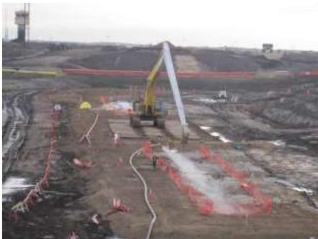
Figure 3. Longstick excavator and slurry being pumped to the Cement Bentonite slurry cut-off wall at Syncrude's Base Mine Dam.
