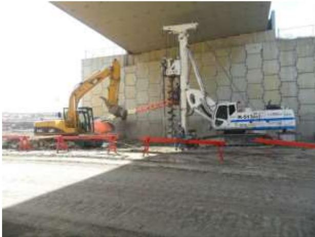
Figure 1. Flight Auger operating beneath Highway 63, Northern Alberta.
