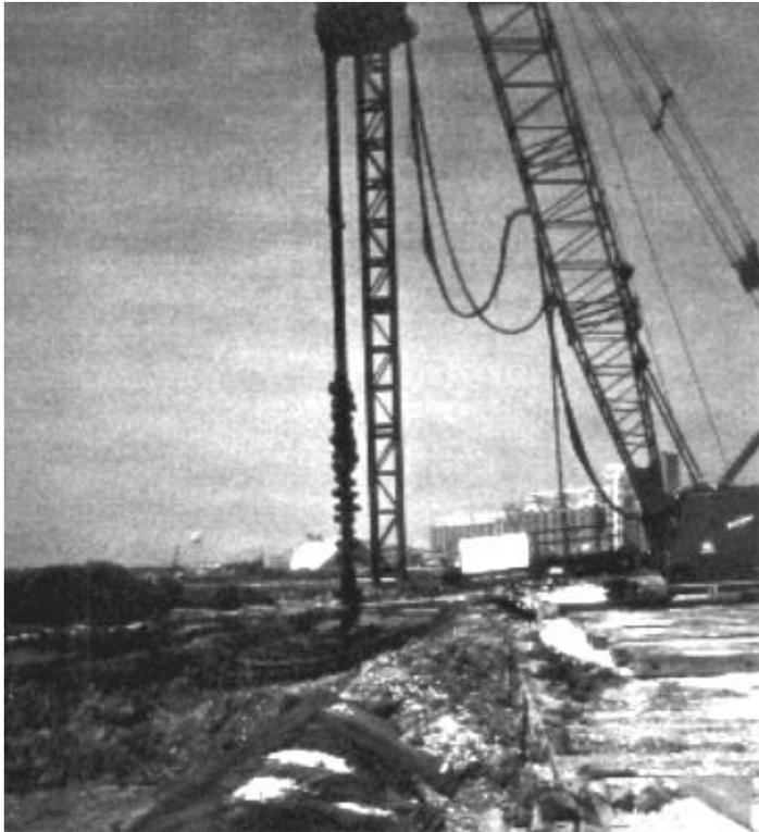
Figure 11. DSM Work in Progress
