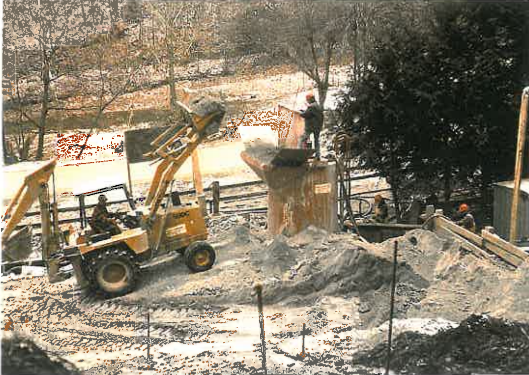
FIGURE 8 - ON-SITE MIXING
