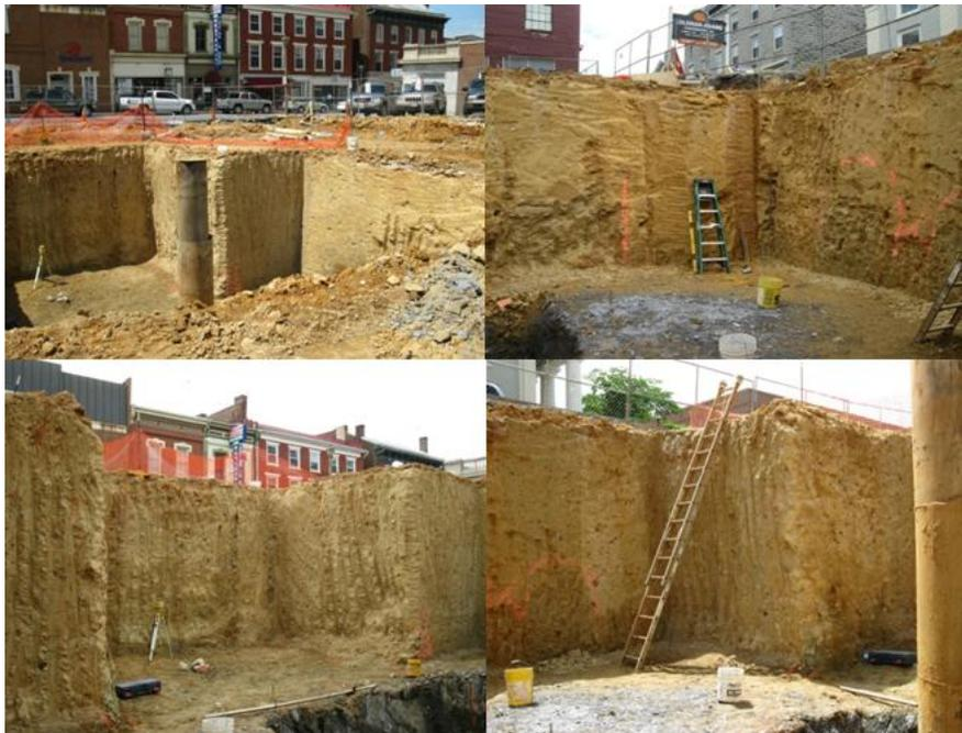
**FIG 4. Pictures of the Excavated Basement Exhibiting the Soilcrete Retaining Wall**
