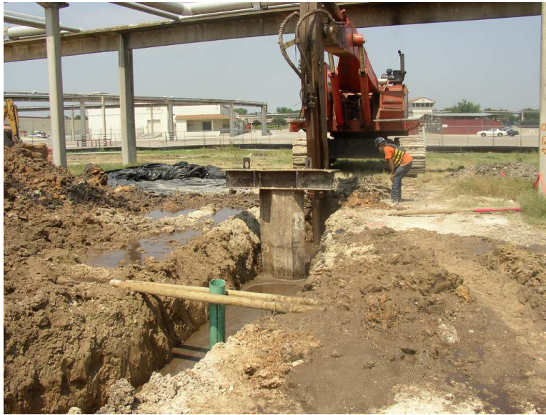
FIGURE 1. Excavating BP trench (note also temporary well and end stop).
