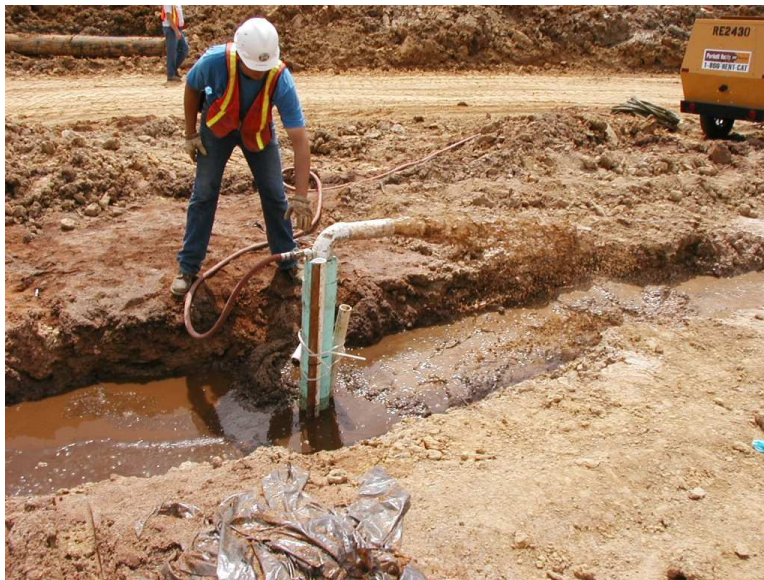
FIGURE 3: Pumping temporary well to break BP slurry and develop PRB.
