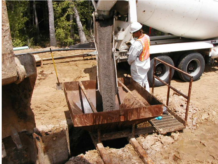
FIGURE 2. Filling tremie from transit mixer.
