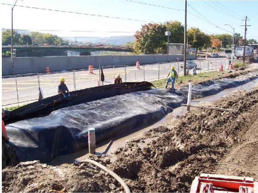
**Figure 4. Liner being placed with overlapped joints**
