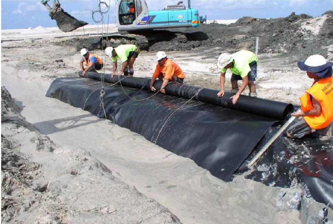
**Figure 6. Placing HDPE panels vertically with overlap**
