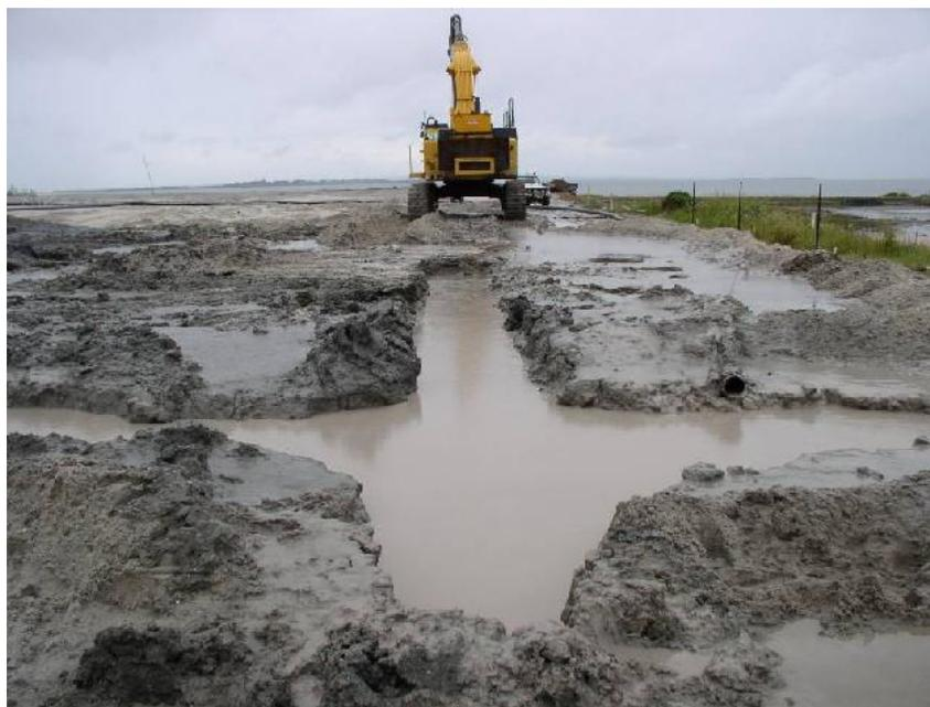
**Figure 5. Excavating the trench supported by bentonite slurry**
