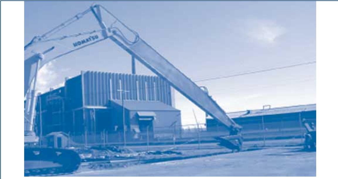
Figure 1. Construction of the extensive PRB trench at the East Helena site required use of a 50-foot-high excavator equipped with a long-reach arm and a 3-foot-wide bucket.
