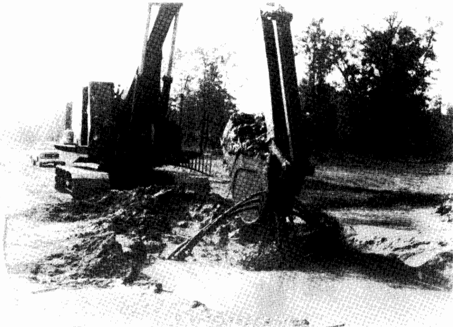
Figure 4 - Slurry Trenching with a Backhoe
