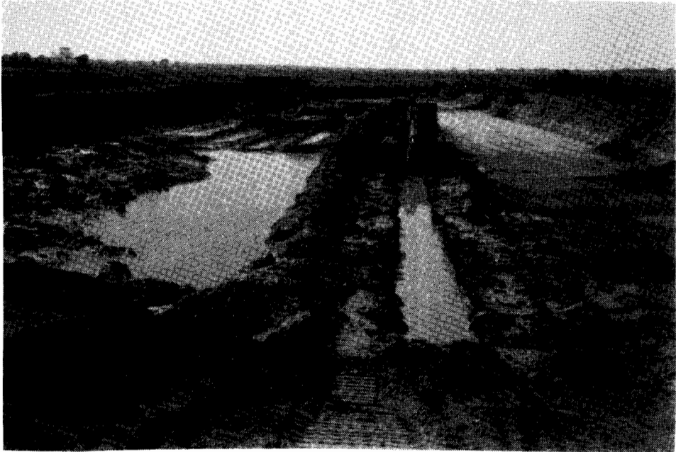
Figure 1 - Trench Excavation and Backfill Mixing Area (Courtesy of Brown & Lambrecht)
