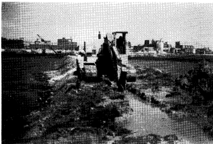
Figure 8 - Trenching Through Construction Dike
