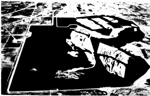
Fig. 3. Aerial view of cooling water reservoir at Braidwood Nuclear Power Station, III.
