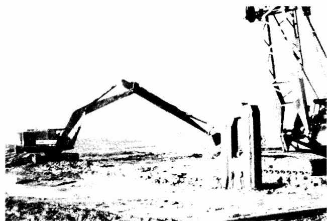
Fig. 9. Equipment used for excavating deep slurry trenches includes a free-hanging clamshell and a modified backhoe capable of excavating to 52 ft. Braidwood Nuclear Power Station, Ill.
