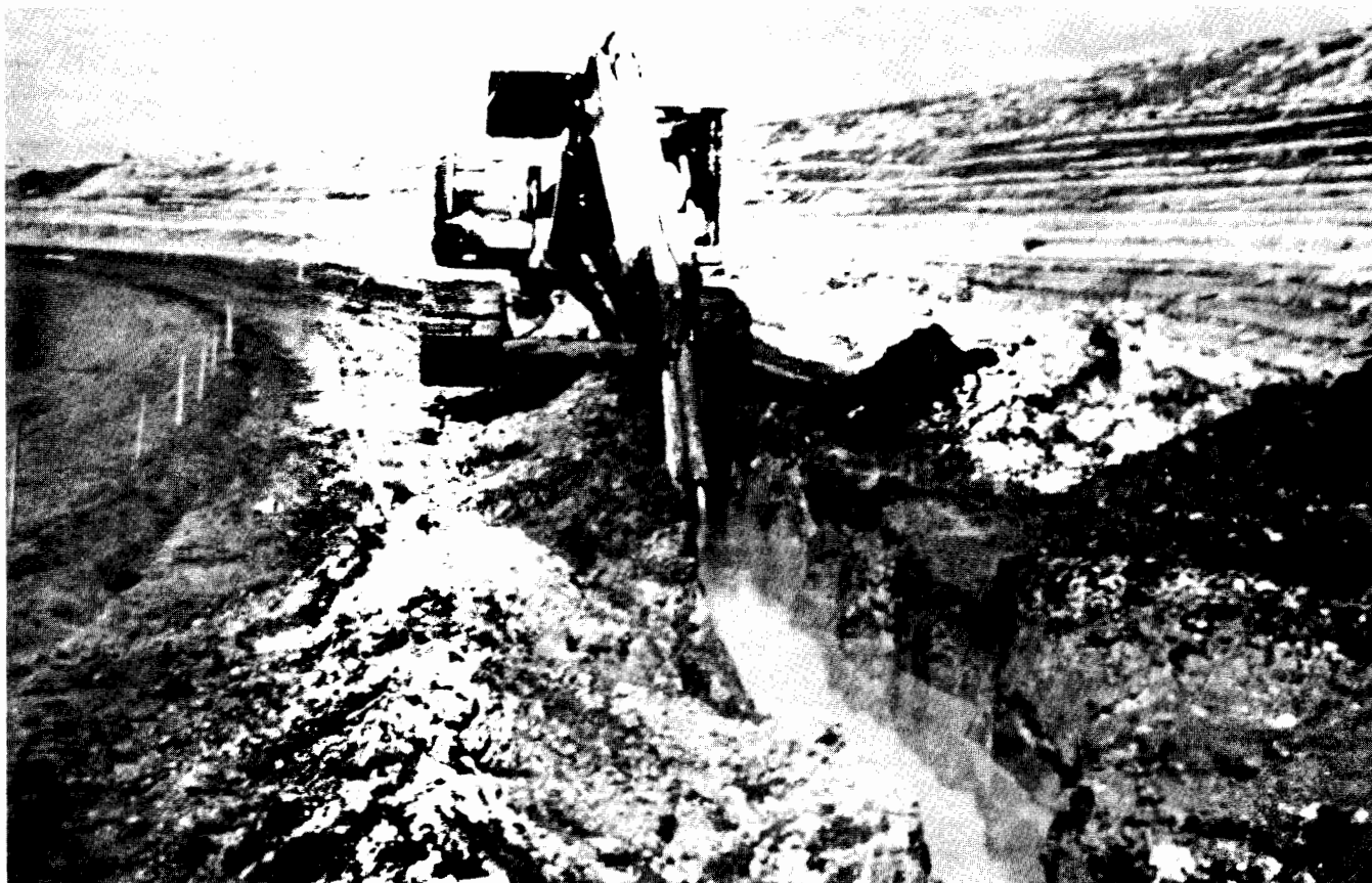
Fig. 1. Constructing cement-bentonite slurry trench along interior toe of slope for cooling water reservoir at Martin Power Plant, Fla. Note soil-cement slope protection in background.
