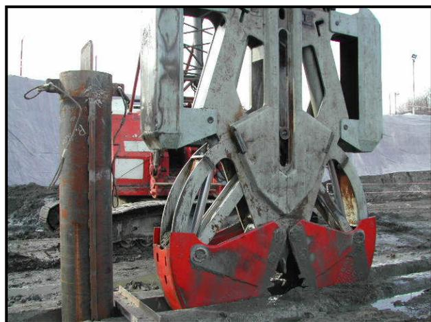
**Fig. 4: Crawler crane equipped and hydraulic grab used in the excavation.**
