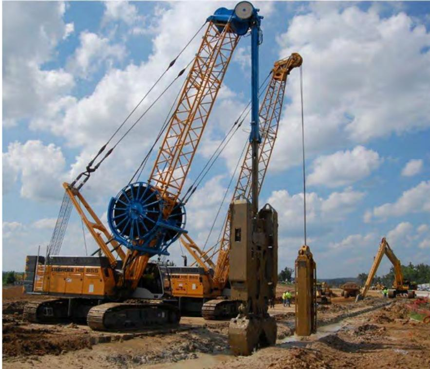
**Fig. 2. Photograph of Clamshells (foreground) and Long Stick Excavator (background) excavating the Smithland Cutoff Wall**
