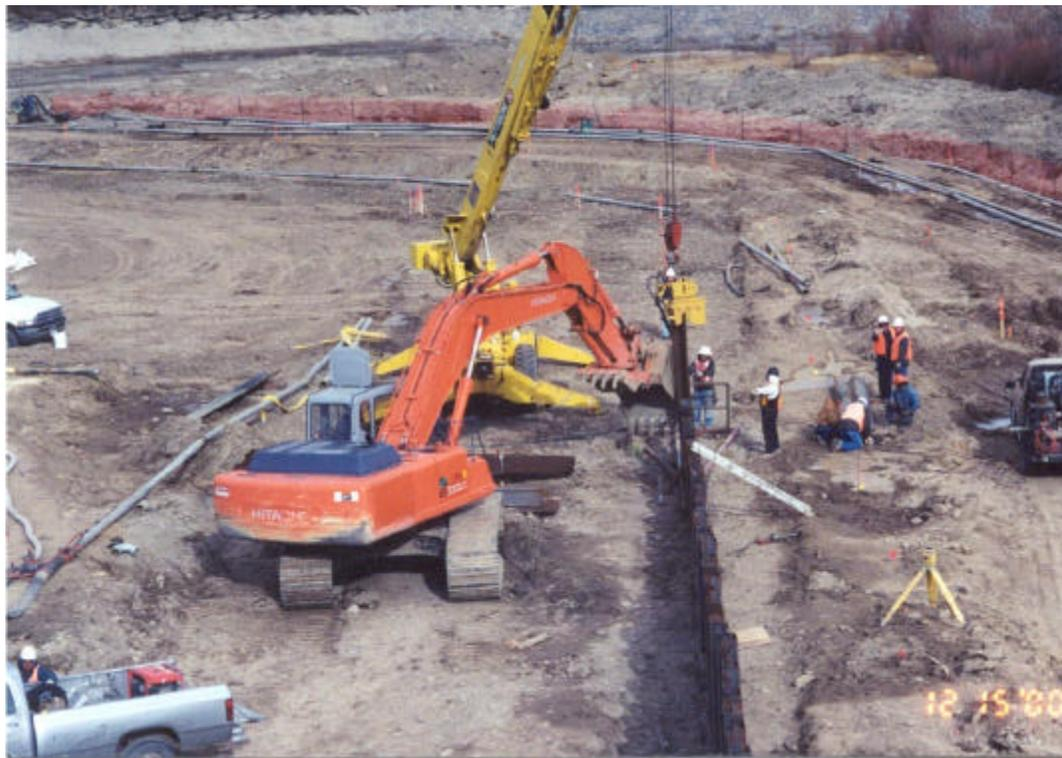
Figure 7: Installation of Steel Sheetpiles in Slurry Trench
