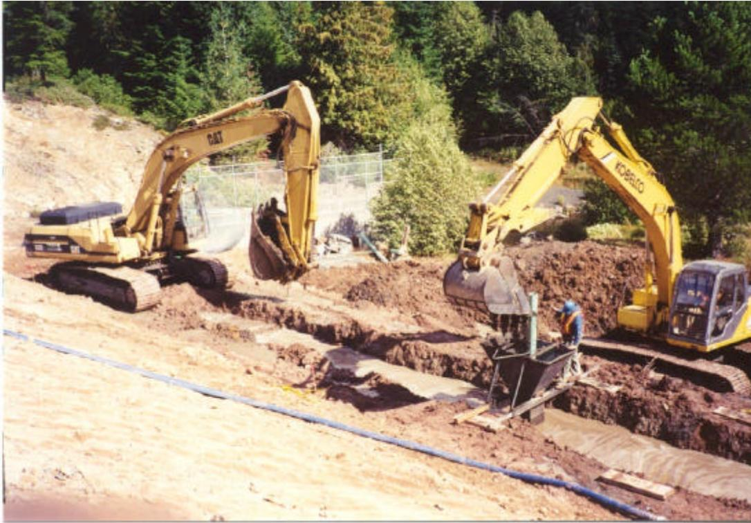
Figure 2: Bio-Polymer Trench Drain Construction
