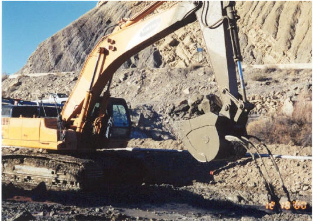
Figure 6: Slurry Trench Excavation of Cobbles and Boulders.
