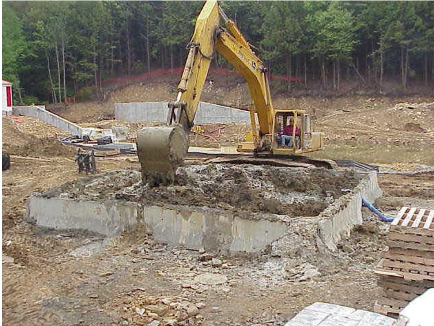
**Figure 3. Mixing SCB Backfill in an Enclosed mixing Area**
