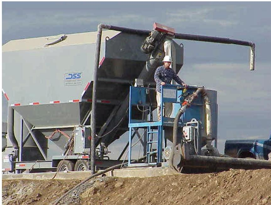
**Figure 4. Grout plant for Mixing Cement Slurry for Addition into SCB Backfill**
