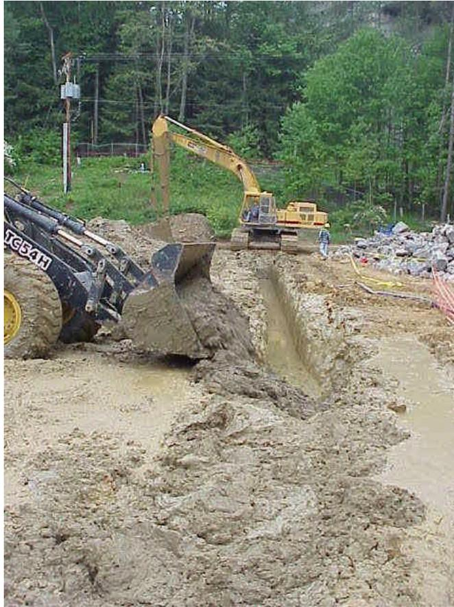
**Figure 2. SCB Backfill being placed in the Trench**
