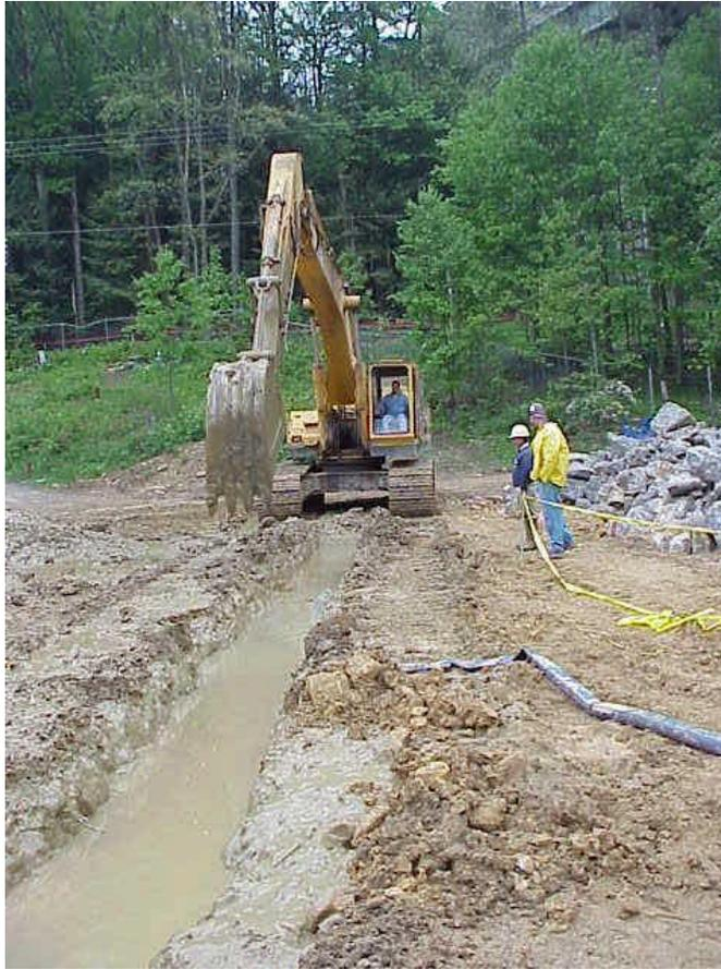
**Figure 1. Trenching Under Bentonite Slurry**
