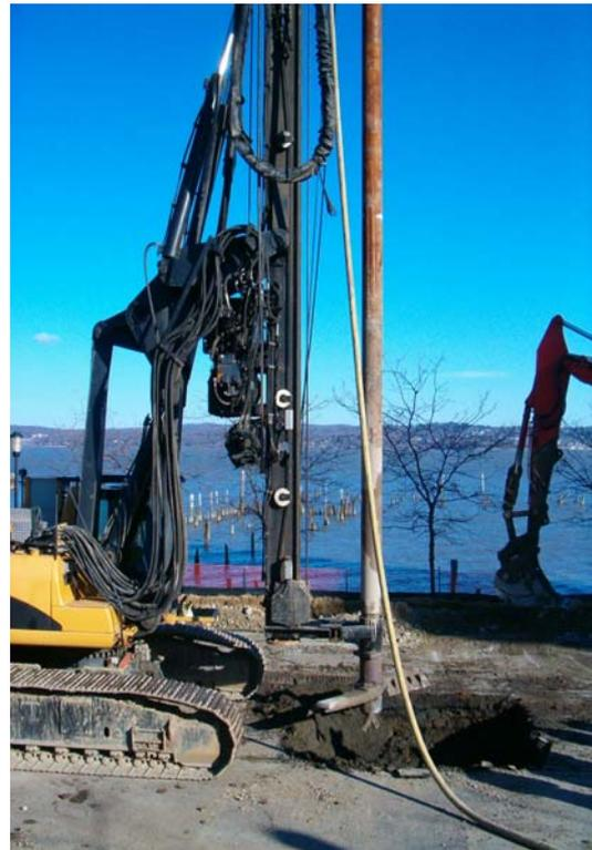
Figure 6: Soil mixing machine with mixer
