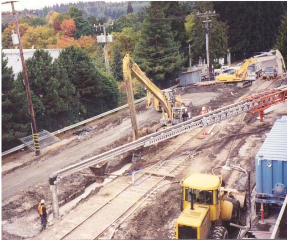
Figure 7: Placing Iron blend In PRB panel in tight site
