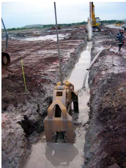
Fig. 1 - Trench excavation for SB wall
