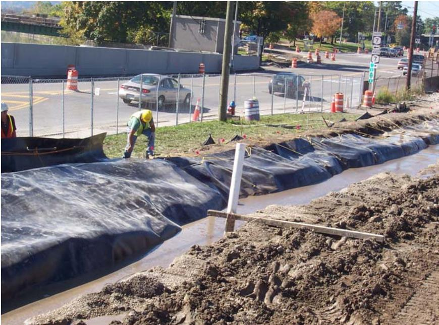
Figure 4: Outer Geo-membrane being placed in slurry-supported trench
