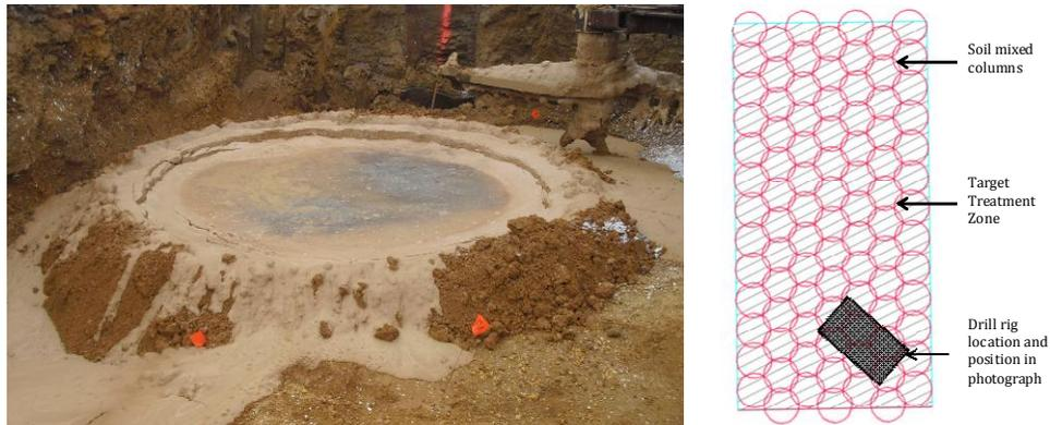
**Figure 2. Treatment of Acetone Impacted Soils in New Jersey**
