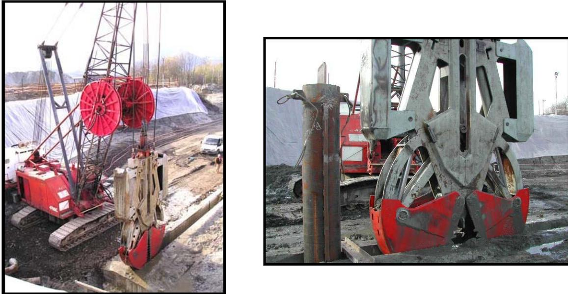
Fig. 5: Crawler crane equipped and hydraulic grab used in the excavation.
