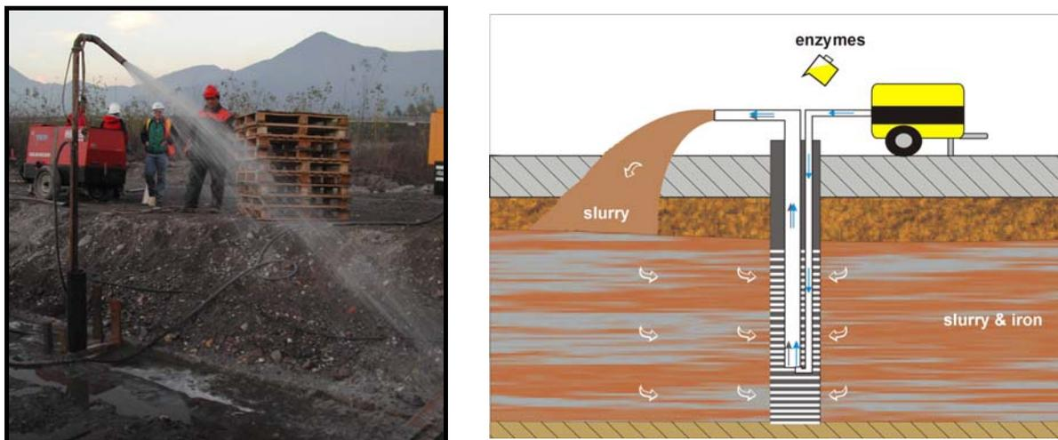
Fig. 6: Degradation of the biopolymer by enzymes recirculation.
