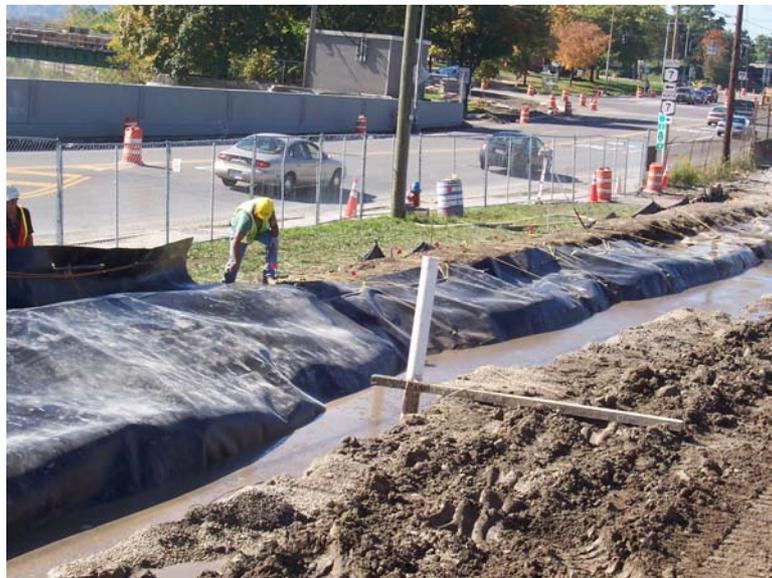
**Figure 5 – Placement of HDPE Barrier**
