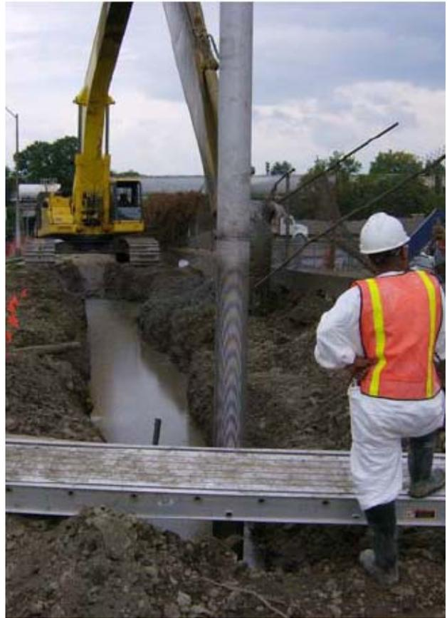
**Figure 4 – Installation of DNAPL Collection Well**
