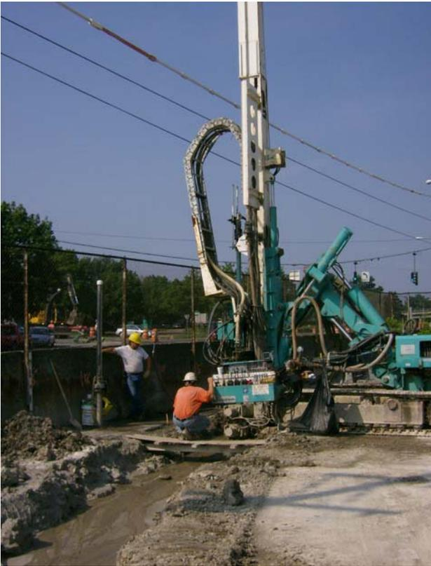
**Figure 3 – Jet Grouting**
