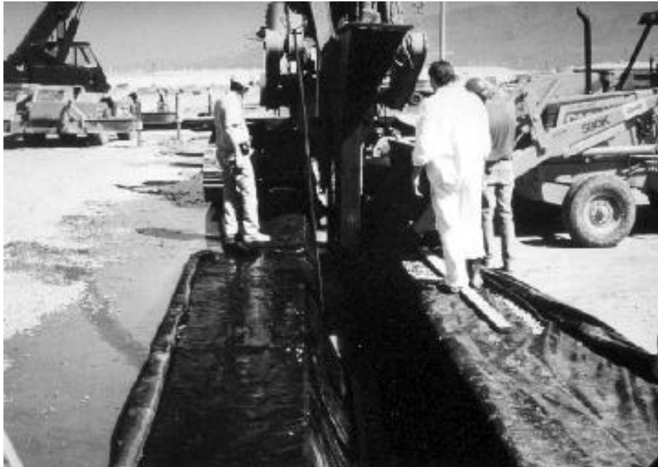
FIG. 5—View of Pipe Installation in Bio-Polymer Trench
