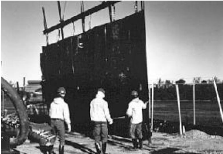
FIG. 3—Installation of Geomembrane Panel
