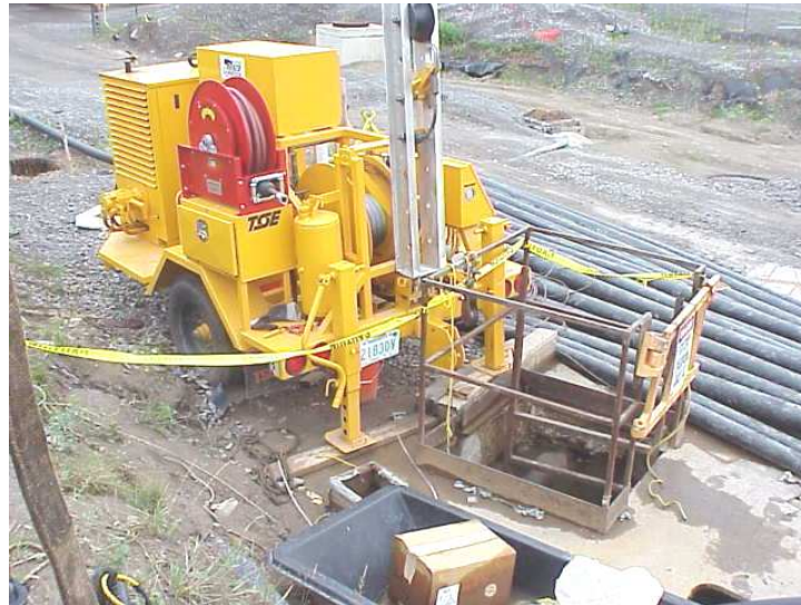
Figure 3. Pipe puller and shaft at the shore end of the project
