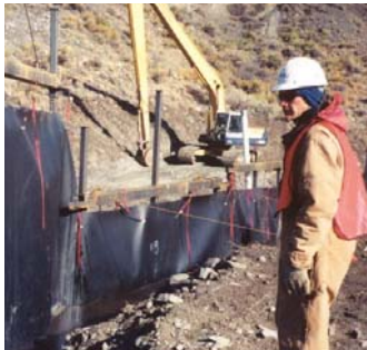
Figure 4: Placing a geomembrane in a BP drain
