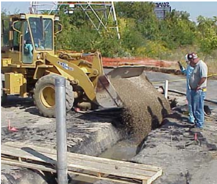
Figure 3: Placing a well and backfilling
