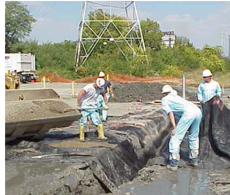
Figure 2: Placing geotextile filter
