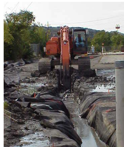
Figure 1: Trenching under BP Slurry
